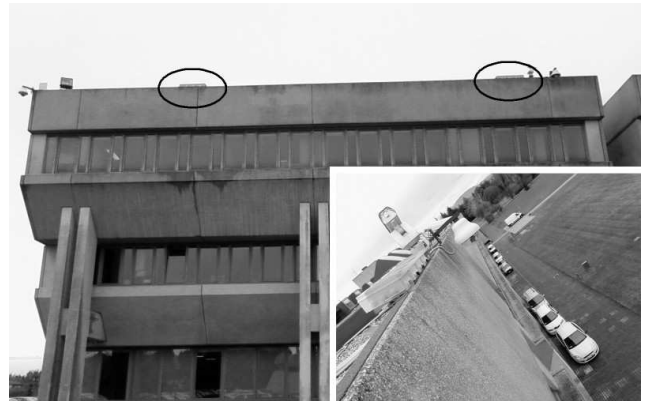
Figure 5: The prototype installed on the roof of the university building. Inside the circles the two arrays. The microphones are protected from the weather by a waterproof box.
